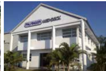
Launch and Recovery Systems Hanoi, Vietnam
