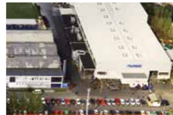
Marine Cranes and Wind Cranes Maribor, Slovenia
